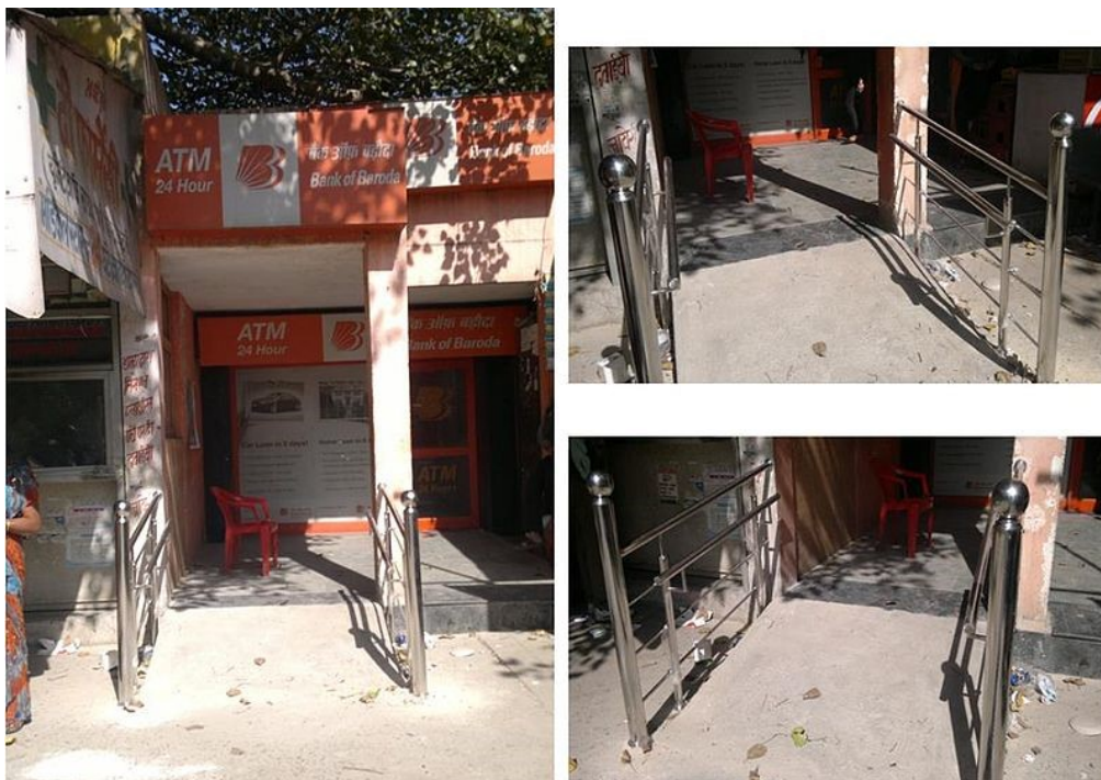
Bank of Baroda ATM in India made accessible by the addition of a ramp. Source: Wikimedia Commons by a CC BY SA 3.0 license.
